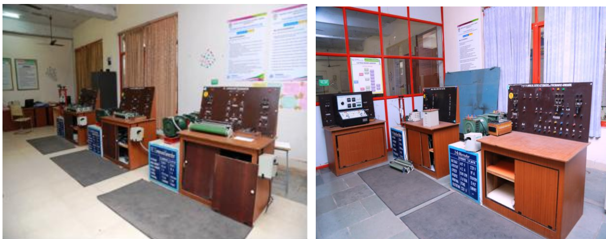
Figure B.6.3 g. Electrical Machines Lab
